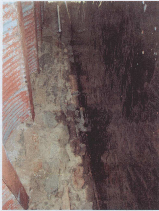
Photo # 2 : General View, Abutment # 1.
